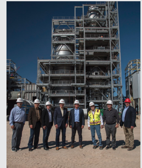
Nebraska Governor Jim Pillen with State and Clean Harbors officials at new Kimball incinerator construction site.
